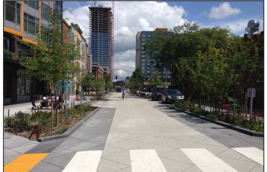
Figure 28. Example of a roadway design that feels more like a pedestrian space vs. a vehicular roadway.
