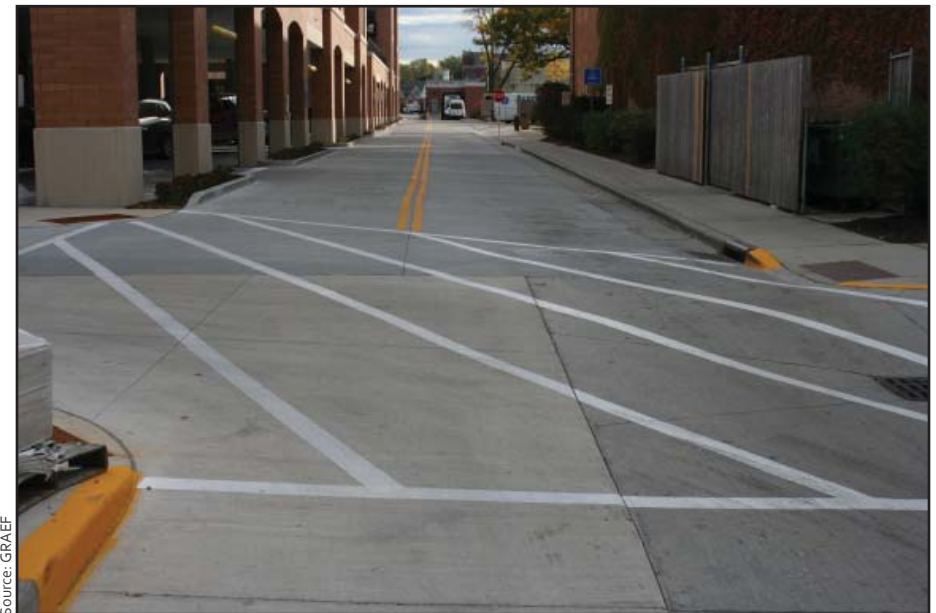
Figure 9. Existing alley condition on the north side of Silver Spring Drive.
